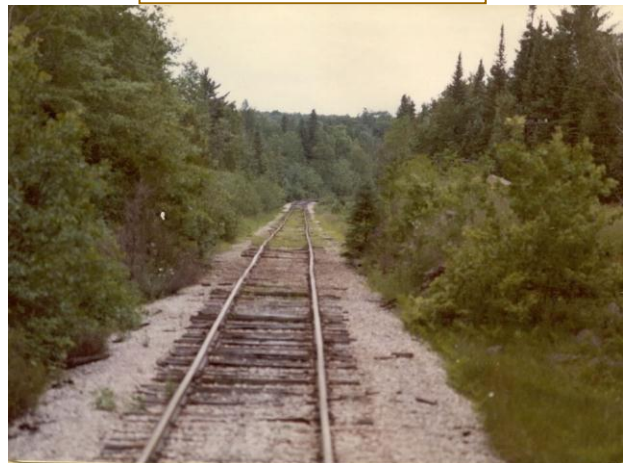
Line Needing Rehab
